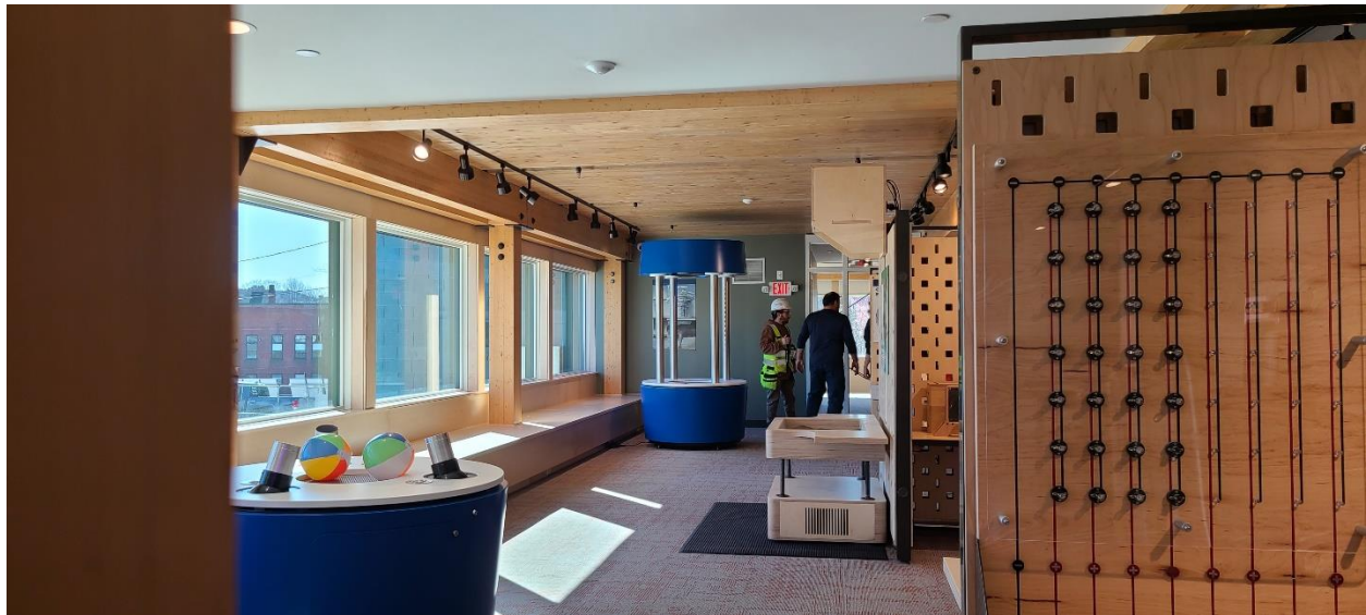
Interior Fairbanks Museum with eastern hemlock CLT exposed ceiling.
